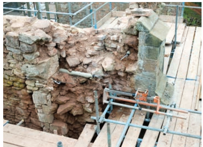
Figure 11 Stitching of fractures
