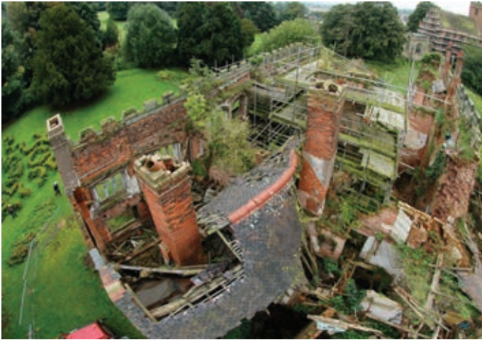
Figure 2 Astley Castle prior to conservation and restoration
