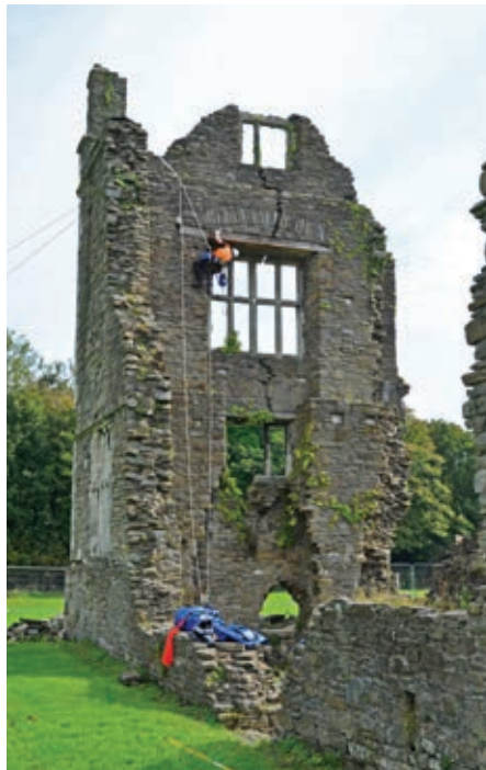
Figure 7 Rope access techniques used to survey Neath Abbey
