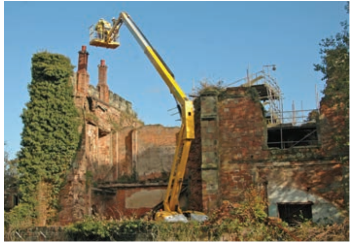
Figure 3 Mobile elevating work platform used to survey Astley Castle
