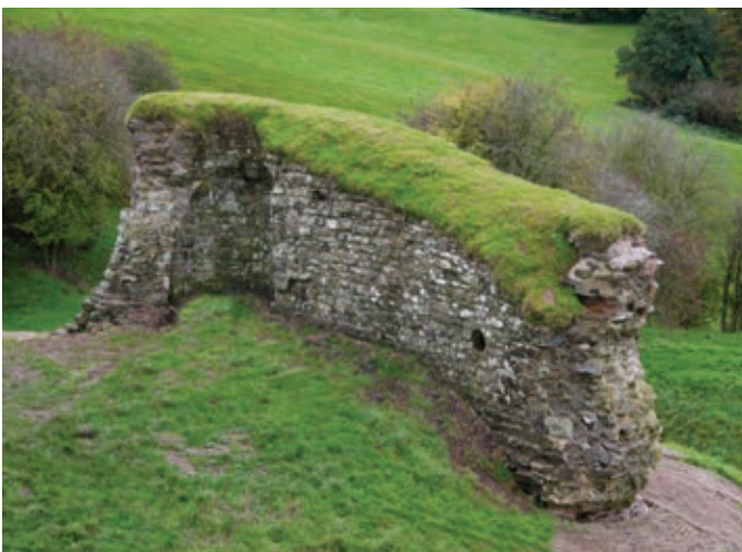
Figure 10 Soft capping works at Kilpeck Castle
